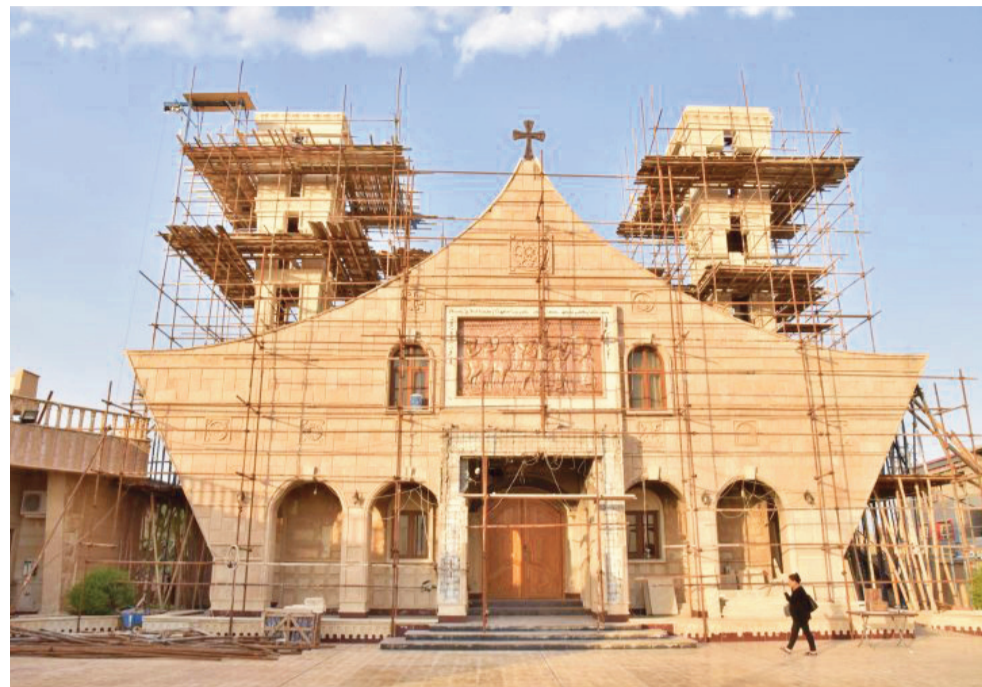
The restoration of the Church's exterior in progress (© ACN)
