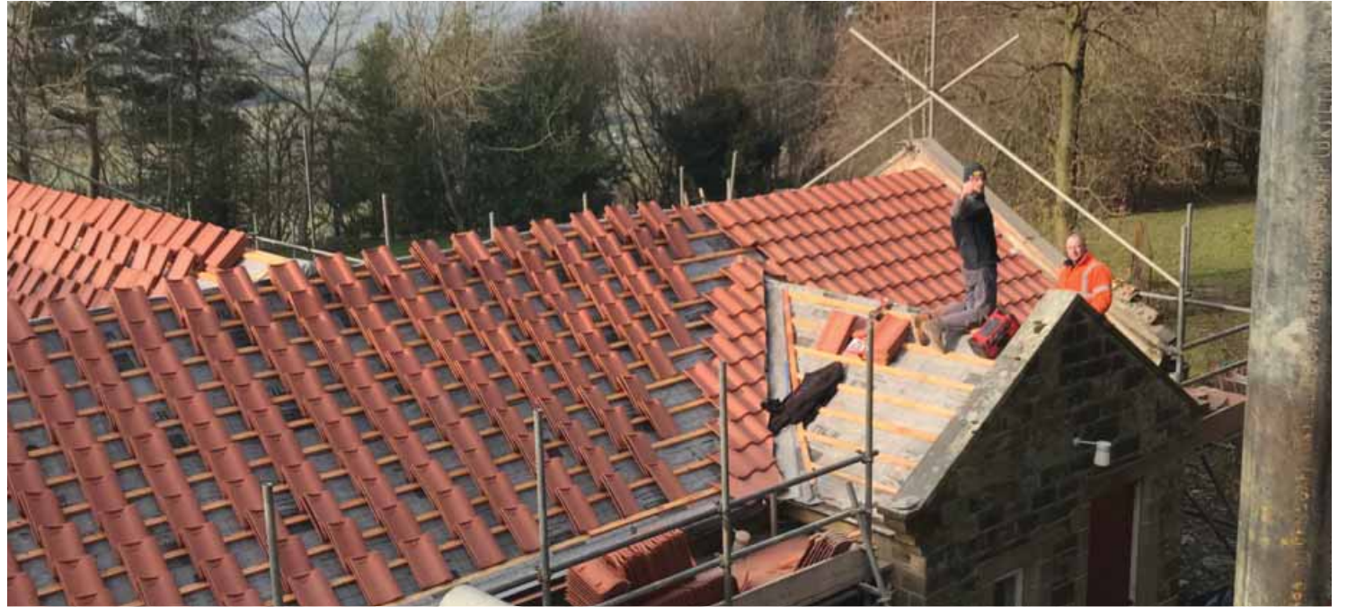
Roofers working on the Lady Chapel and hall
