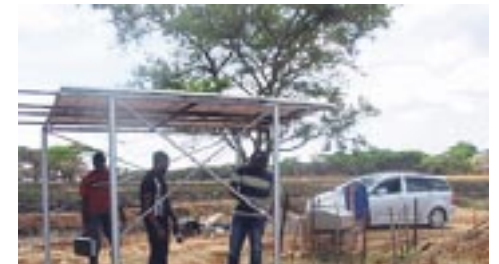
The solar pump up and running just three weeks after appeal was launched
