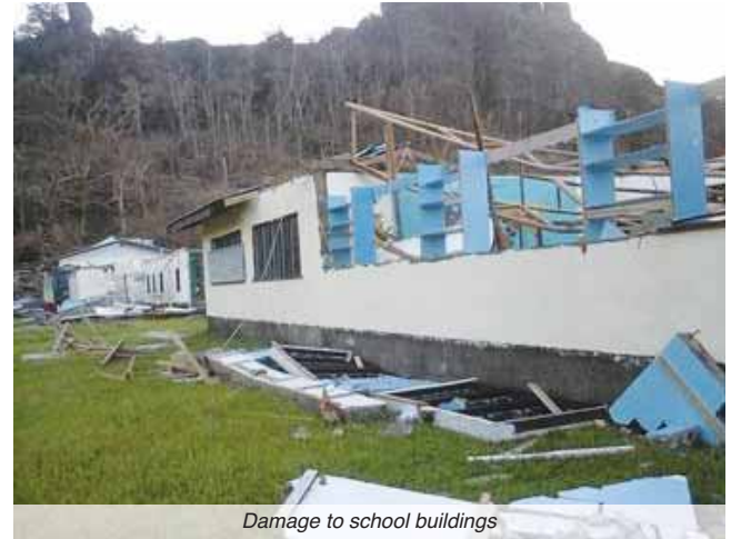
Damage to school buildings
