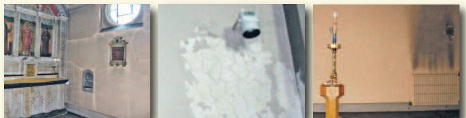
Close-ups of the deterioration
