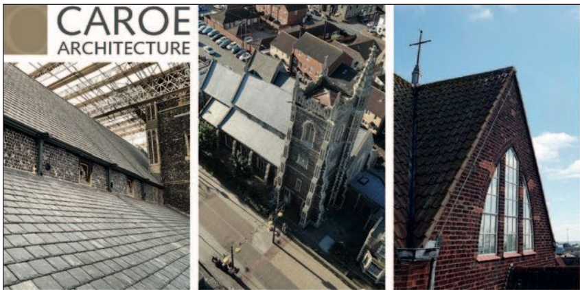
Roof Detail of St Mary's, Great Yarmouth
