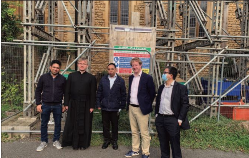
DECEMBER 2021: MP Paul Bristow (second right) visited St Peter and All Souls church in Peterborough which needs to raise £1.3 million to deal with major subsidence issues which are threatening the church structure.
